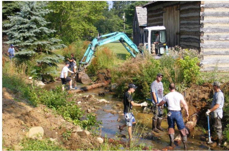
Stream Restoration Preserving Property Value of 1798 Compass Inn in Laughlintown
