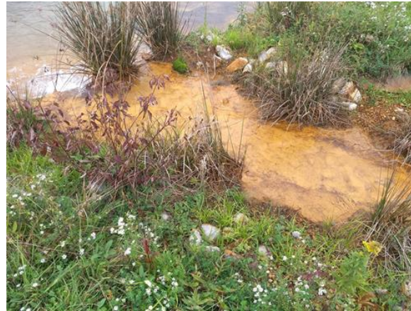
Kalp Discharge Remediation at Indian Creek Credit: Anna Perry
