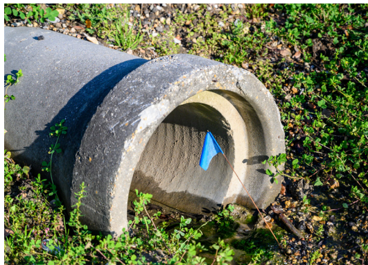
MCM #3 under the MS4 program requires regular screening of stormwater outfalls to detect any illicit discharges.
