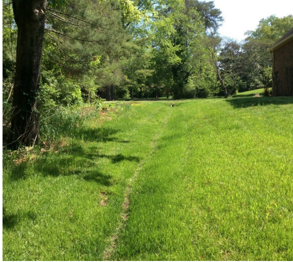
Grass swales (above) are a structural BMP that can help mitigate the effects of stormwater once a site has been developed.
