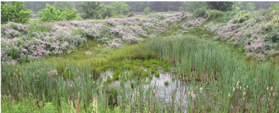
Constructed wetlands remove pollutants, and reduce peak flow rates and runoff volume.
