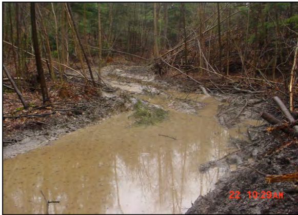
Improperly constructed logging road with poor drainage allows water to collect and sediment to enter the nearby stream.
