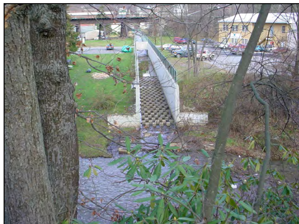
Tanners Run, a tributary to Anderson Creek, is enclosed in a concrete channel in Curwensville.
