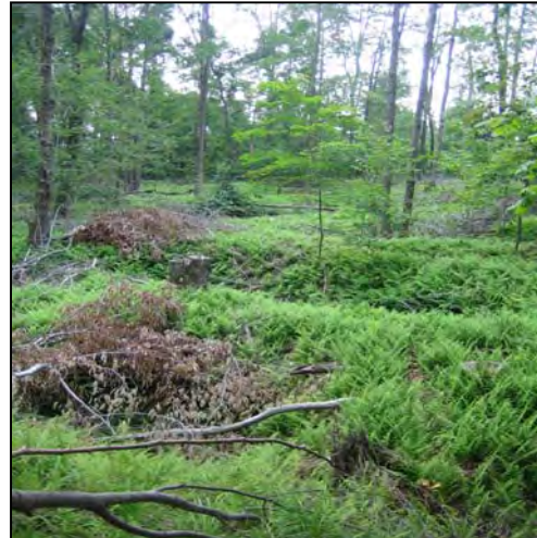
Subsidence area above the Spencer clay mine. Note the numerous depressions. Such areas direct rain and surface water directly into the underground mine, which increases pollution. Subsidence areas are extremely hazardous to nearby residents.
