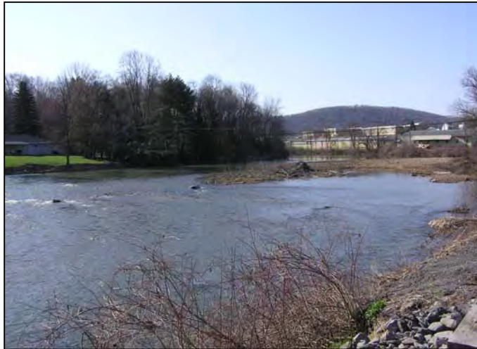
Gravel bar, which has formed in the West Branch of the Susquehanna River at the mouth of Anderson Creek, is causing erosion along the streambank in the background.
