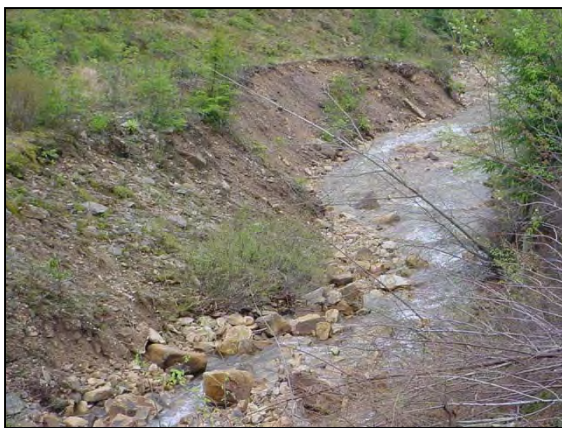
Large erosion site on Bear Run, immediately below the water-supply reservoir.
