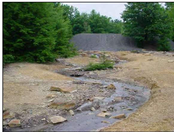
Combined Korb2 and Korb3 discharges draining into an unnamed tributary to Anderson Creek (UNT AC8.2).
