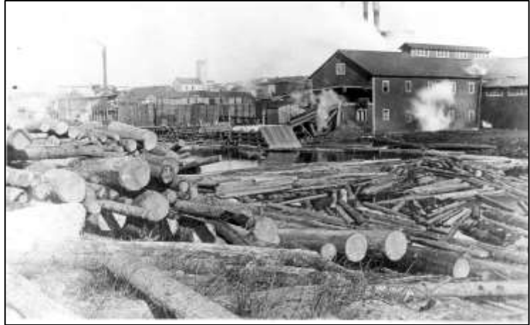
Figure 4. Babcock lumber mill. Source: Western Maryland Historic Society
