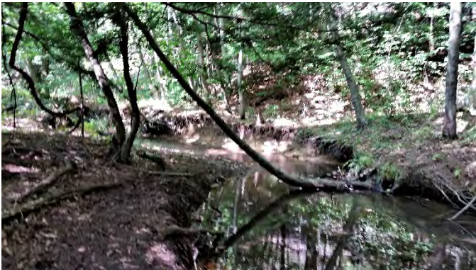
Bank erosion along Little Brubaker Run
