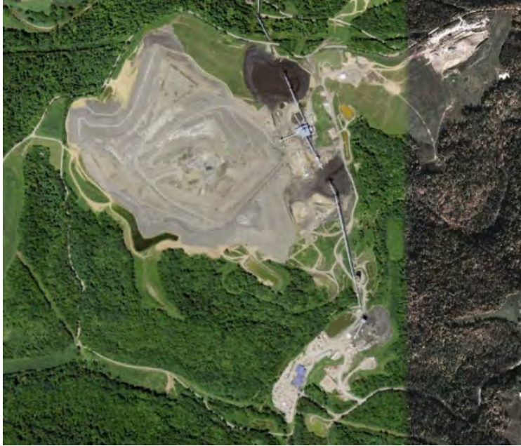
Figure 118. Located in Wayne Township, the AEC Century Mine has multiple NPDES discharges that are regularly monitored by the Ohio EPA for compliance within pollution limits, including mine water, sanitary wastewater, and industrial stormwater (OEPA 2010). Water quality parameters for Century mine discharges remain within NPDES requirements and the permit currently has no defined limits on discharging total dissolved solids (Wood-Pugh, personal communication, 2011). Photo source: “American Energy Corporation - Century Mine.” 39°53’43.88” N and 81°01’21.17” W. Google Earth. October 27, 2011. October 22, 2012.
