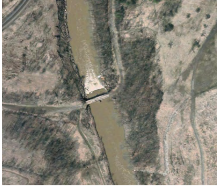
Figure 132. An abandoned bridge across Captina Creek (RM 5.5) in Section 21 of York Township partially obstructs flow and may be a barrier to fish movement upstream. The bridge serves as access to abandoned gravel pits from State Route 148. Photo source: Google Earth.
