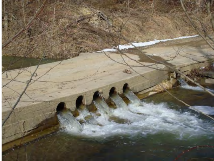
Figure 130. Located in Washington Township, this low-water bridge crossing Joy Fork is a barrier to fish migration upstream (OEPA 2010). Source: Belmont Soil & Water Conservation District.
