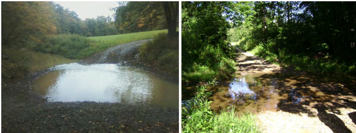
Figure 111. Public and residential stream crossings for vehicles, including these township roads located in the Bend Fork subwatershed ( left , Goshen Township) and the Piney Creek subwatershed ( right , Washington Township), can contribute to sedimentation downstream. Photo sources: Belmont Soil & Water Conservation District, 2012 and 2013.
