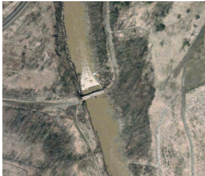
Figure 93. A 20-foot culvert passes under this access bridge across Captina Creek in York Township.
