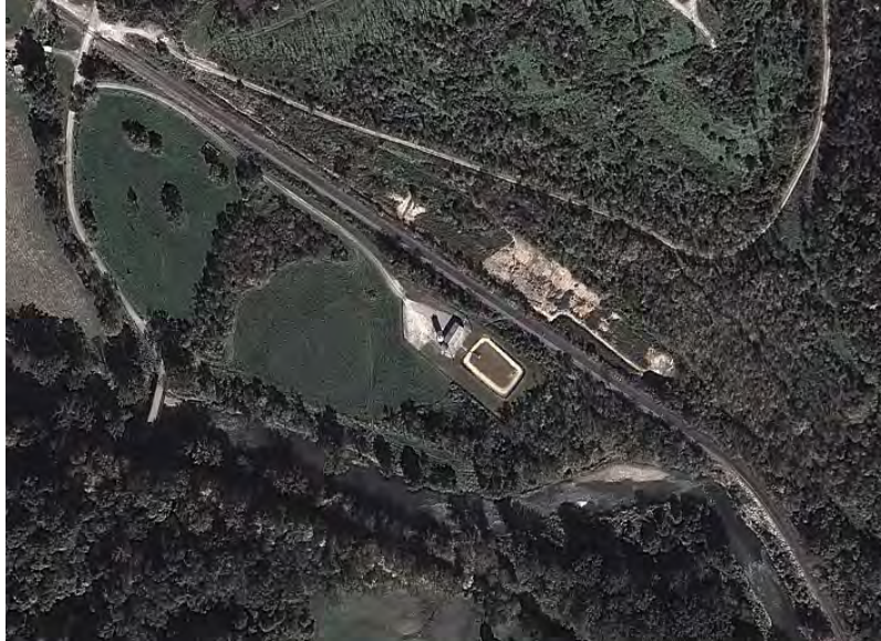
Figure 127. Located in the Pea Vine Creek subwatershed, Bellaire Corporation's Powhatan No. 5 coal mine in central York Township has been reclaimed and an NPDES permit requires monitoring for stormwater runoff and AMD seepage. A dosing silo and settling pond treat acidic water pumped out of abandoned mine shafts with alkaline material before it can enter Captina Creek. Additional reclamation is planned by North American Coal, the current owner of the site. Map source: "Town Run Reclamation Site." 39°52'51.32" N and 80°50'31.08" W. Google Earth. October 7, 2011. December 27, 2012.
