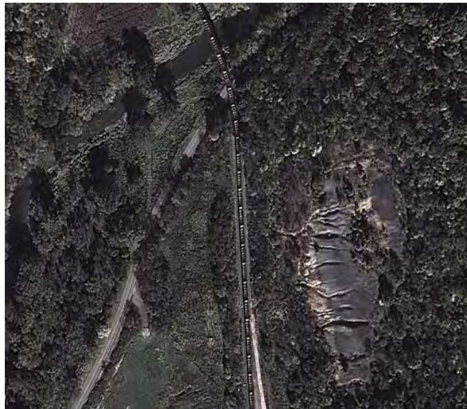
Figure 124. Located in Section 4 of Washington Township (Pea Vine Creek subwatershed), a portion of the gob pile at the Linn Tipple facility between State Route 148 and the railroad tracks was recently reclaimed by Murray Energy. A large area remains on the hillside east of the railroad tracks and leaches AMD into a roadside ditch along State Route 148, but effects on water quality downstream are minimal. Map source: “Linn Tipple Gob Pile.” 39°54’04.93” N and 80°54’18.76” W. Google Earth. October 7, 2011. December 27, 2012.
