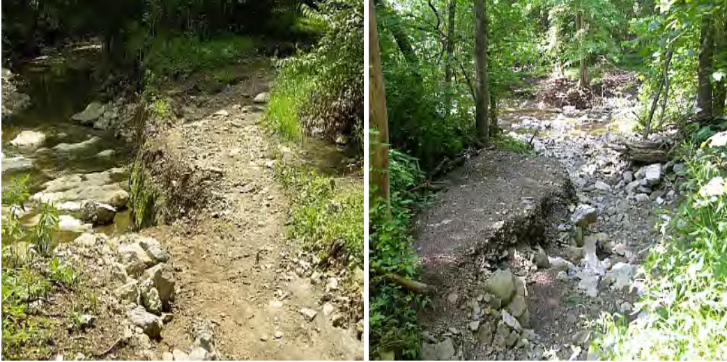
Figure 112. (Left and right) Anderson Run, in the Pea Vine Creek subwatershed. ATV traffic on abandoned township roads along this tributary has accelerated rates of erosion on exposed streambanks, resulting in increased sedimentation downstream. Photo source: Belmont Soil & Water Conservation District.
