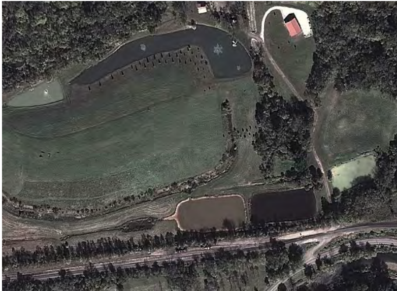
Figure 123. Settling ponds surrounding the reclaimed Cravat Coal gob pile, located in the Pea Vine Creek subwatershed. AMD from the pile is passively treated with limestone slag before entering the creek. Officials from Ohio Department of Natural Resources – Division of Mineral Resources Management (ODNR-DMRM) have stated that creating passive treatment wetland habitat around the edge of the gob pile would further decrease the threat of AMD entering the stream from this location. Map source: “Cravat Coal Reclamation.” 39°53’36.67” N and 80°53’28.36” W. Google Earth. October 7, 2011. October 22, 2012.
