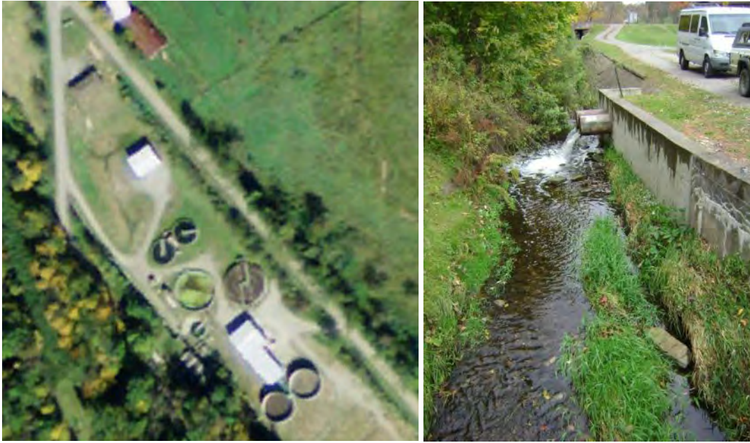
Figure 113. The Barnesville waste water treatment plant ( left ) after completion of 2011 upgrades. Treated discharge enters the North Fork of Captina Creek ( right ). Map source : “Barnesville Waste Water Treatment Plant.” 39°58’12.54” N and 81°09’45.75” W. Google Earth . October 27, 2011. October 22, 2012. Photo source : Belmont Soil & Water Conservation District, 2012.
