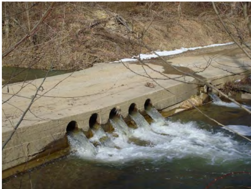
Figure 78. A fish barrier formerly located on Joy Fork, within the Bend Fork subwatershed (OEPA 2010).
