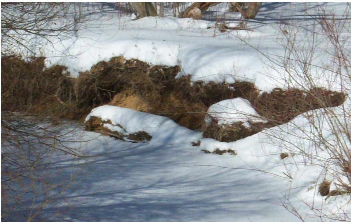
Figure 90. – Close up view of slumping banks, lower section of headwaters tributary of Chest Creek (looking upstream)
