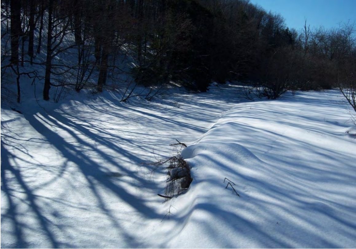
Figure 68. – Minimized sediment transport, lower end of impaired segment, mainstem of Chest Creek (looking upstream)
