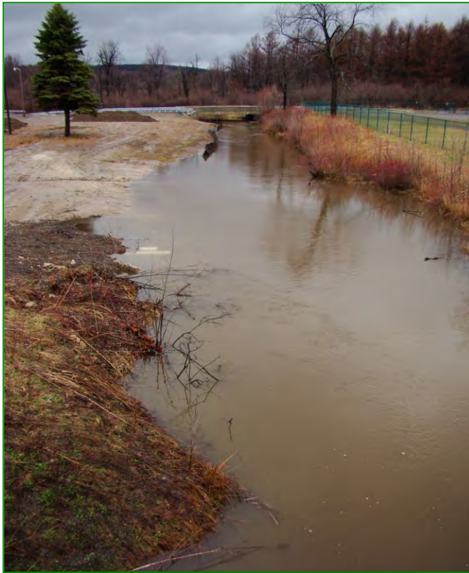
Figure 22. Clear Shade Creek near State Route 56 bridge with a marginal riparian rating. Photo by Melissa Reckner.
