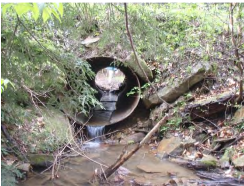
6203: Perched culvert on private access road (left), three pipes on relic logging road (right).
