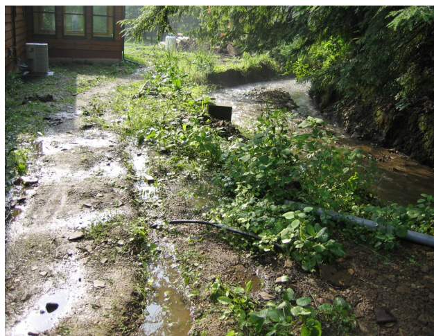
Figure 7: Soil disturbed by construction erodes at extremely high rates and is easily washed into streams by precipitation.
