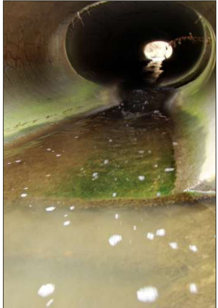
Figure 26. Culvert in the headwaters of Rocky Run Photo by Melissa Reckner
