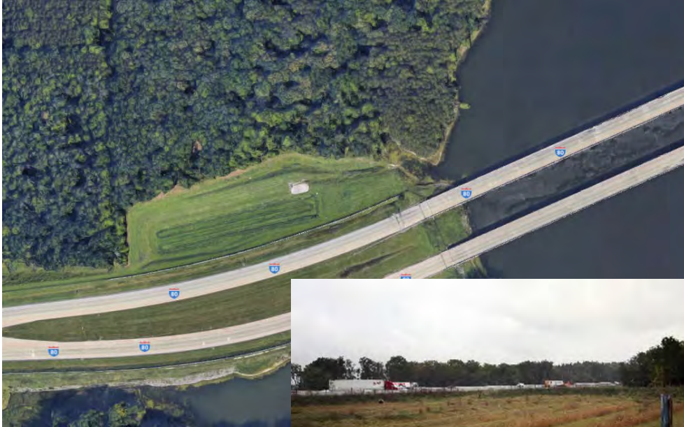
Photo 1: Aerial view of Westbound Meander Reservoir Spill Containment Basin
