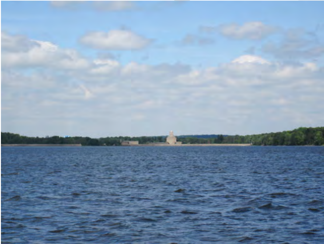
Meander Reservoir Dam with Meander Water Gatehouse in the background
