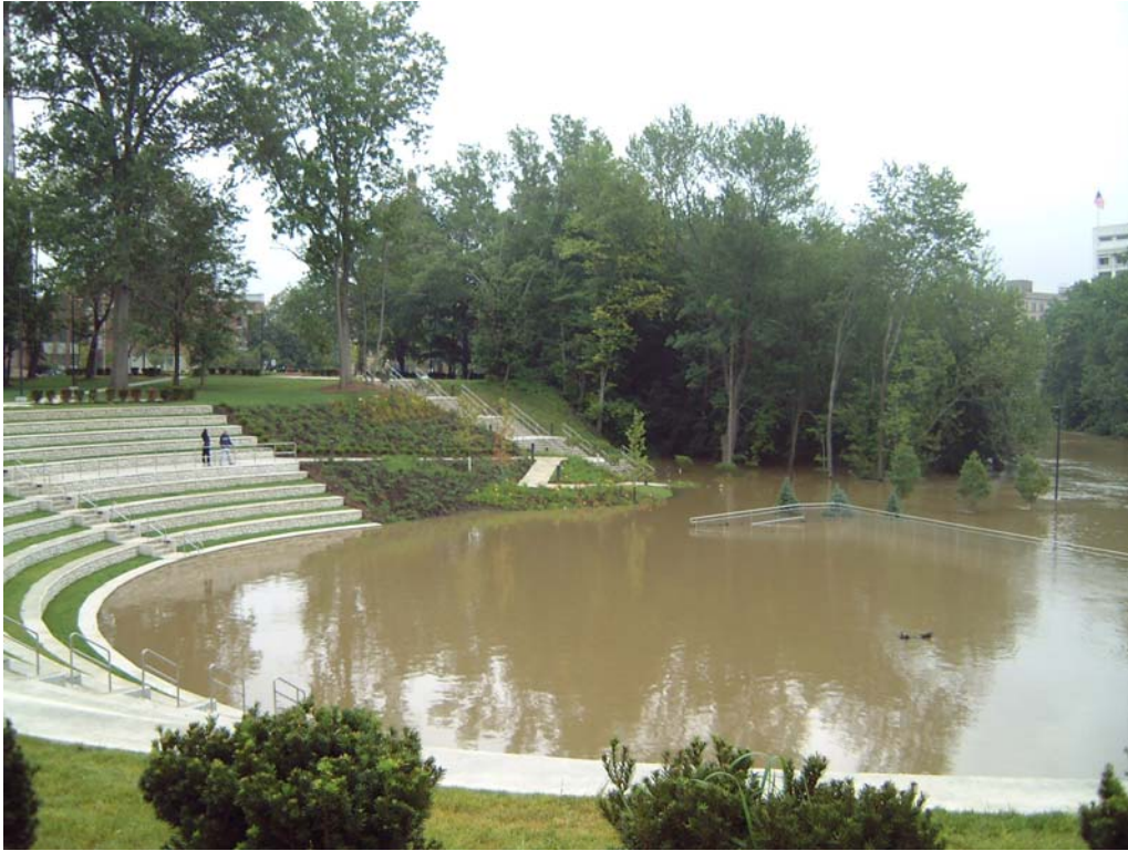
Figure 4-8. Flooding in Perkins Park Ampitheatre, Warren, OH, July 23, 2003 (photo by T. Nuskievicz).
