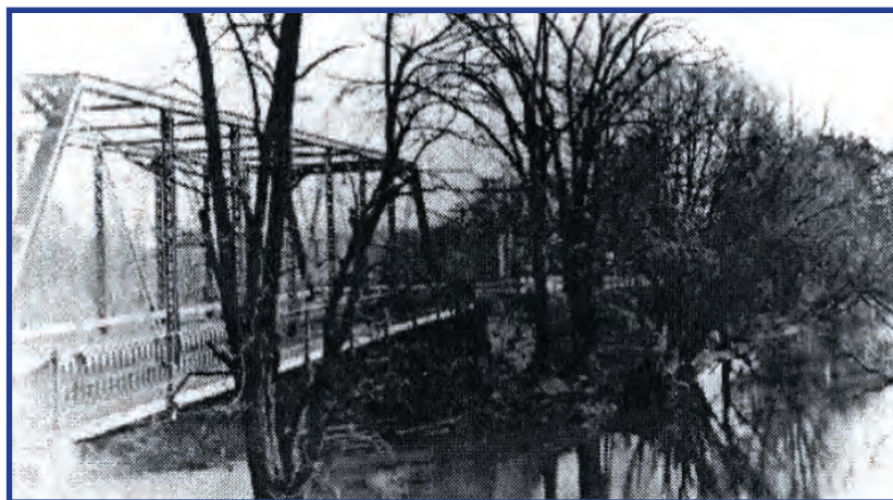
Iron bridge over Pymatuning Creek in Kinsman. Courtesy of the Trumbull County Historical Society
