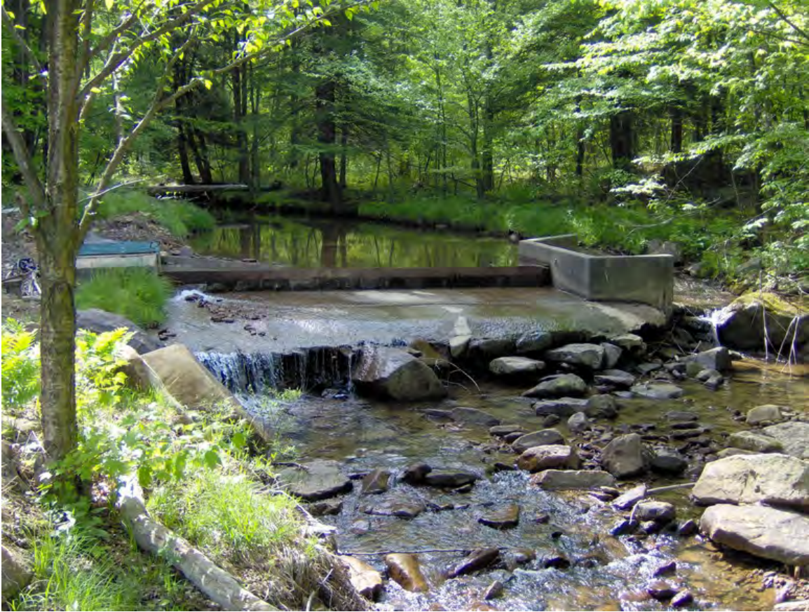
Dam in stream for Westover Municipal Authority
