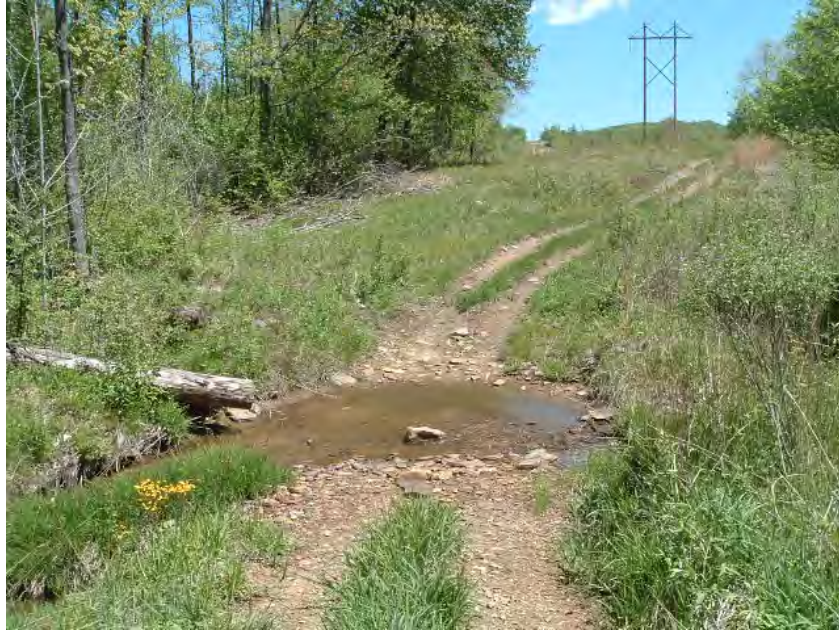
Powerline with road
