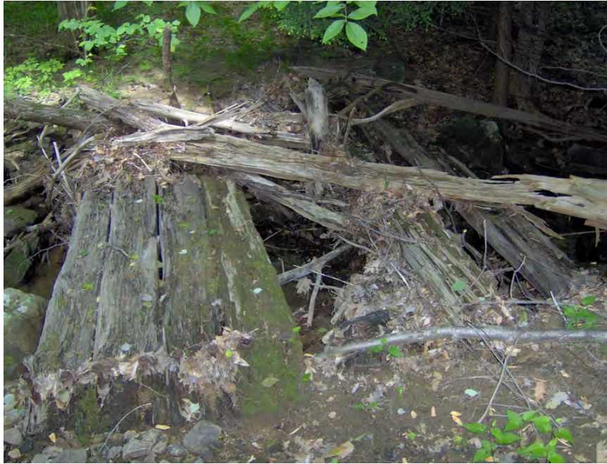
Old bridge located on the pipeline tributary.
