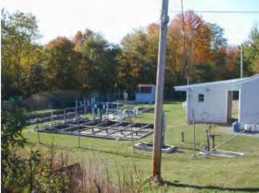
Clintonville sewage treatment plant.
