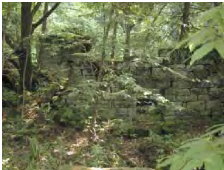
Old Scrubgrass Mill located near the mouth of Trout Run
