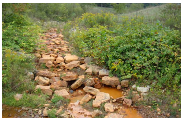
Figure 4. Reclaimed abandon mine drainage swale into Glens Run, 2010.
