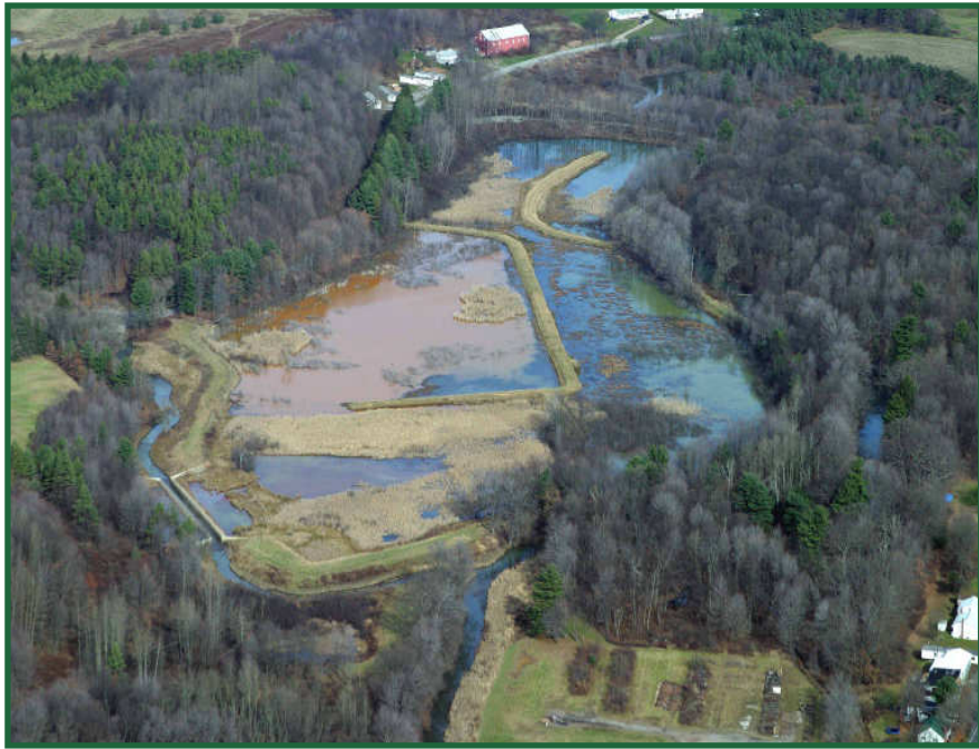
An aerial view of the Boswell Passive Treatment System.
