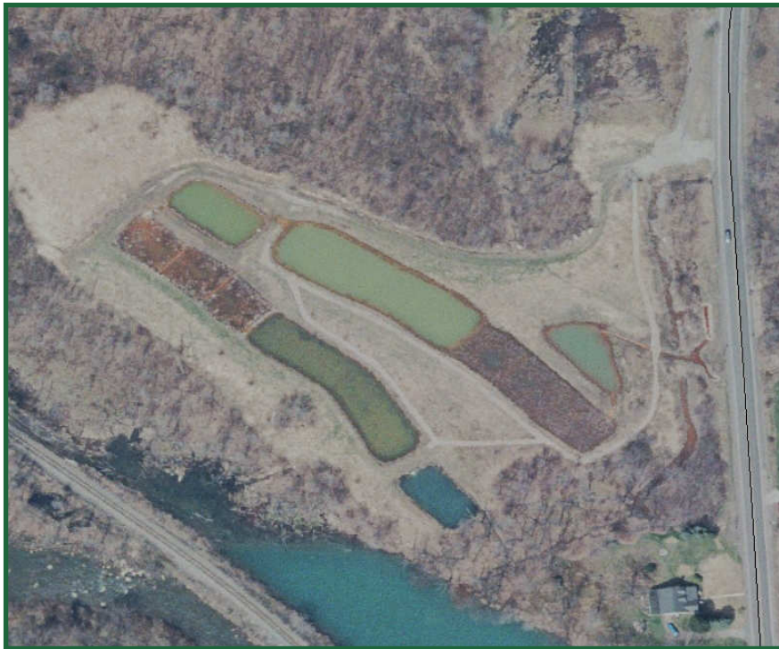
(Left) Site D of the six-site Oven Run Passive Treatment system as seen from an aerial photograph.
