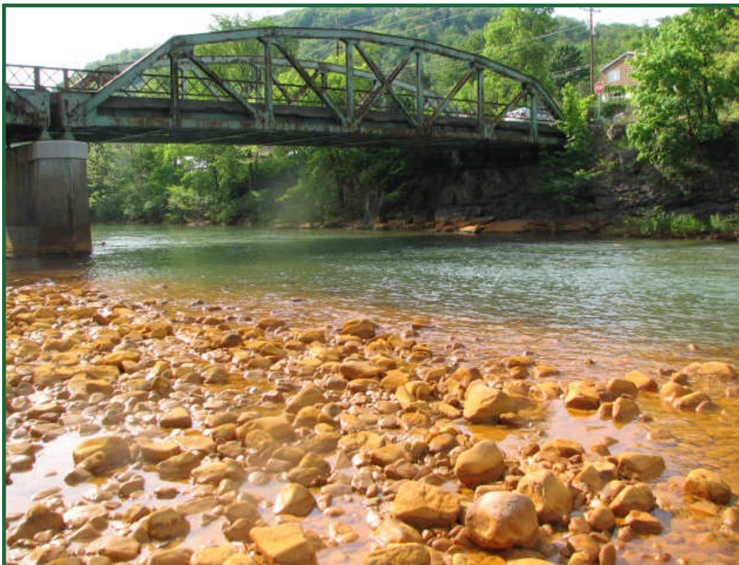
The orange coloration on rocks in the Stonycreek River at Krings shows the visible effects of abandoned mine drainage.
