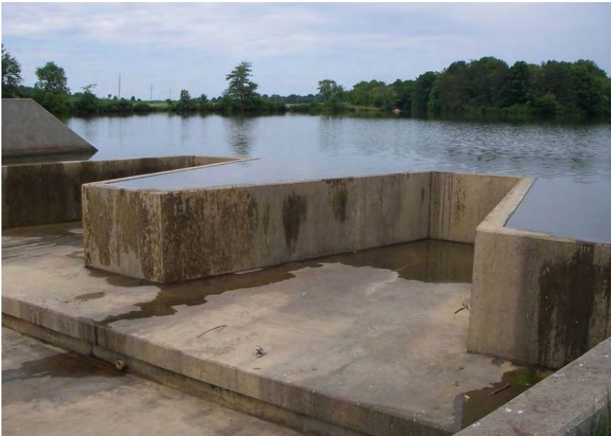
Figure 18. Overflow structure for Westville Lake showing zero discharge conditions on July 3, 2007 (photo by Chris Hunt, Ohio EPA).
