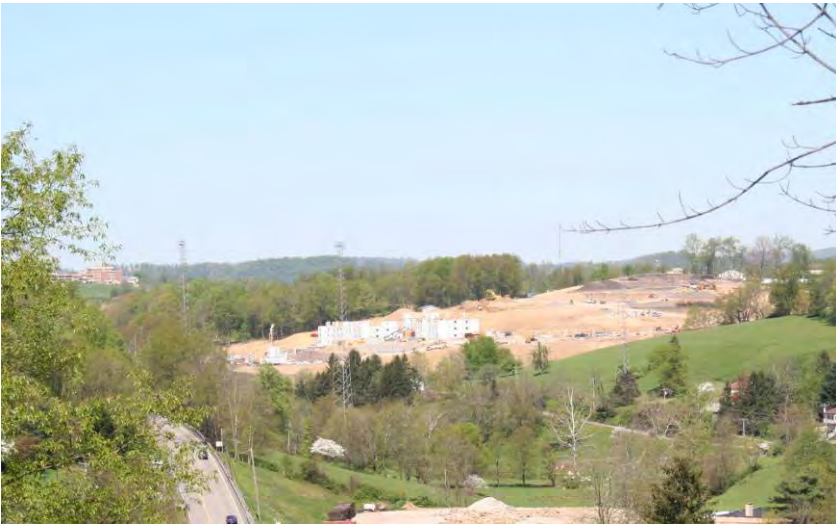
Figure 26: Development above the poorly constructed retaining wall.
