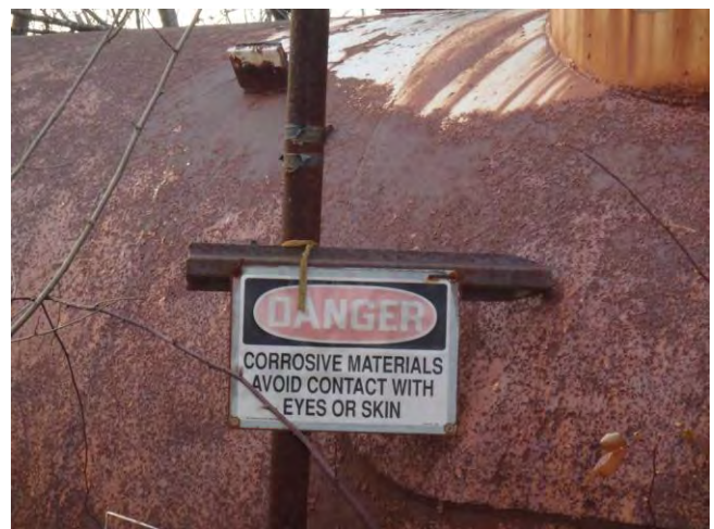
Abandoned caustic soda tank on abandoned mine lands.
