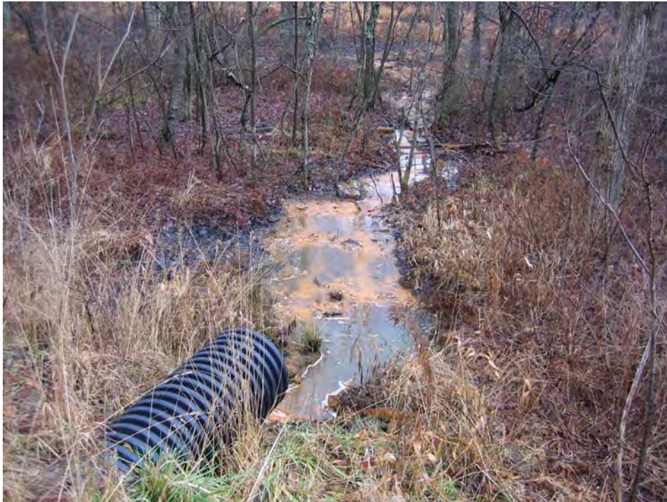
Figure 15; County Road 53 Bridge, Source 2
