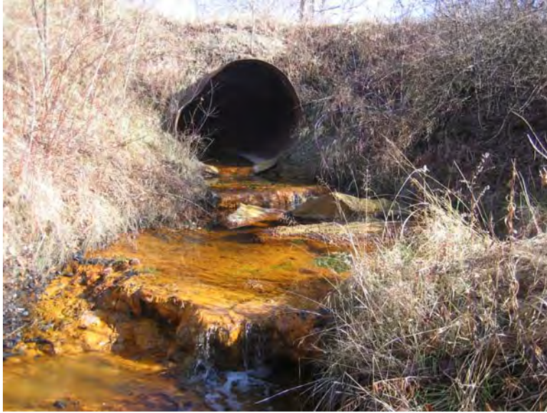
Figure 7; Wolf Run Culvert Source
