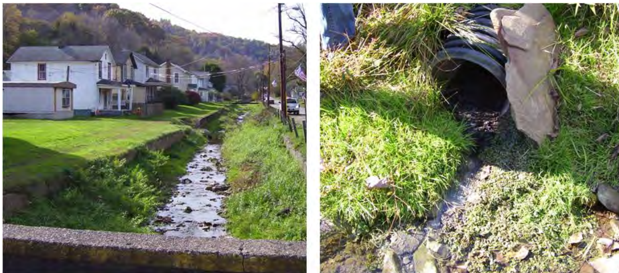
Figure 7.2. Homes along a tributary to North Fork Yellow Creek in the unsewered community of Irondale (left). Storm sewer with a suspected sewage discharge (right).
