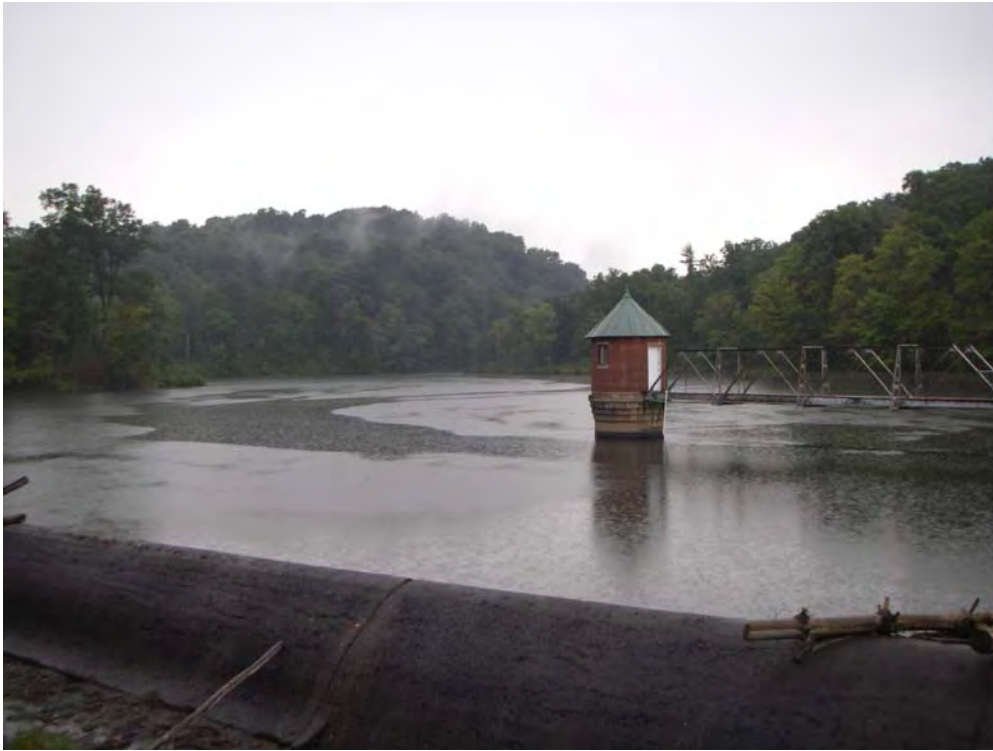
Figure 7.3. Wellsville Reservoir and Buckeye Water District intake photo taken from spillway 9/6/06.
