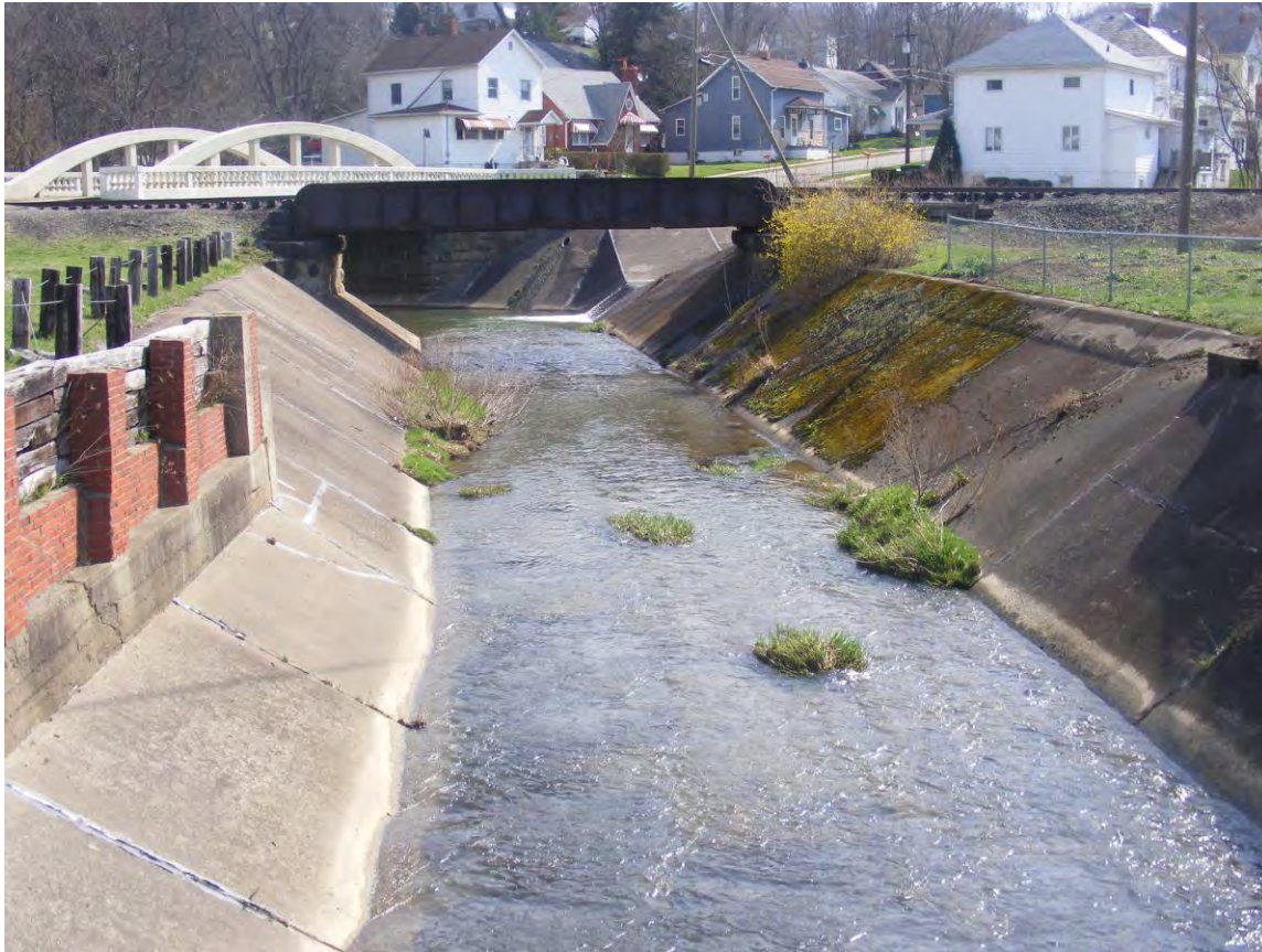
Fig. 42: The mainstem of Yellow Creek channelized through the village of Amsterdam (Corder)
