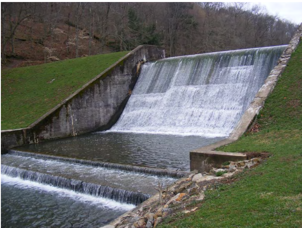
Fig. 108: Spillway at Jefferson Lake State Park
