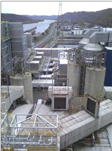
Fig. 14: FirstEnergy Sammis Plant Tour (Corder)
