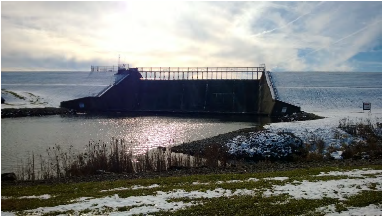
Evans Lake Spillway (Source: Eastgate)
