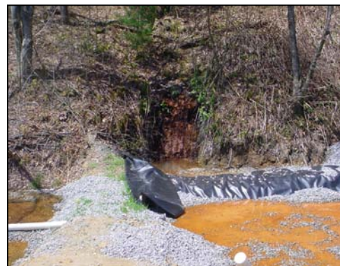
Photo of WR5 Treatment System
