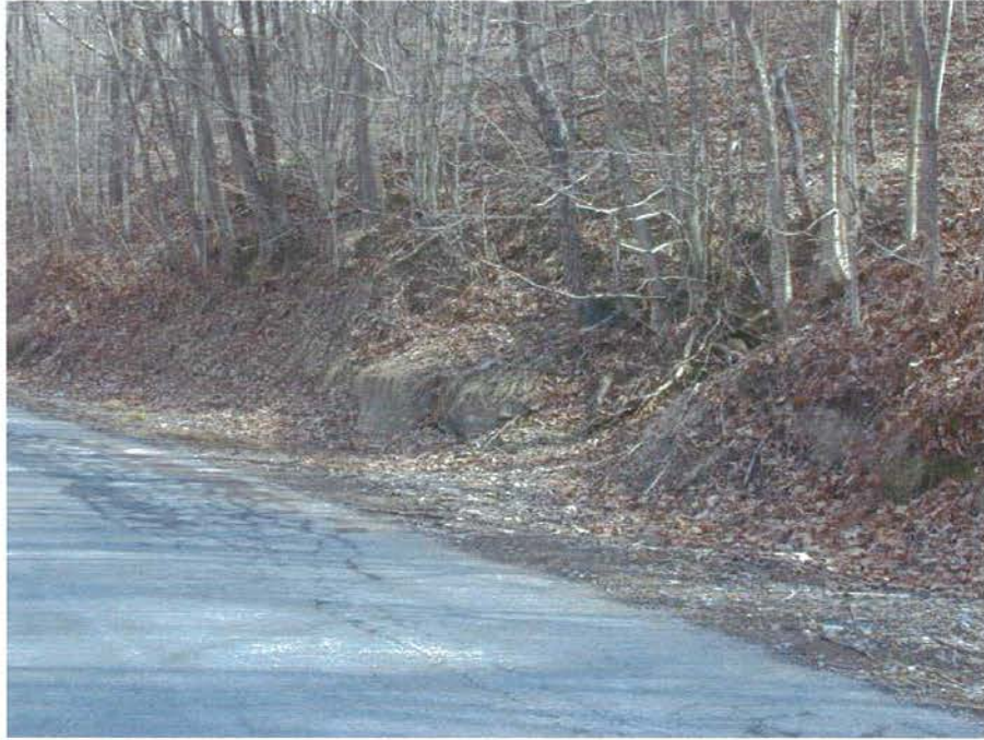
Figure 7. Hillside erosion contributes sediment to the Rudolph Run watershed.
