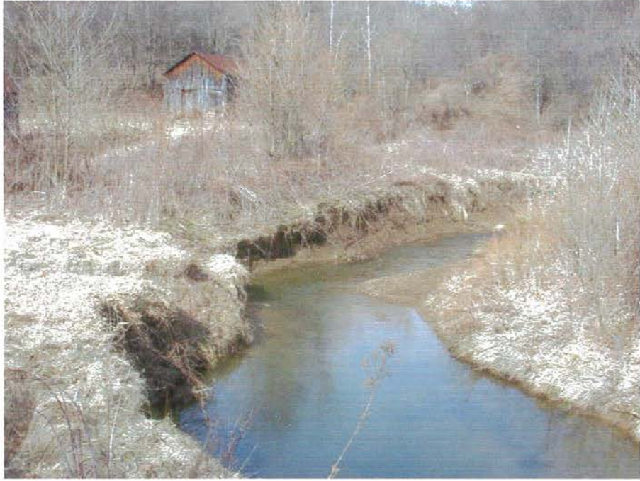
Figure 5. Bank erosion in the lower Rudolph Run watershed.
