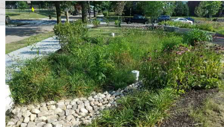
Tåsinge Plads - Copenhagen's first climate change-adapted urban space; storage allows sewers to handle larger cloudburst storms (Source: DHI Group)
