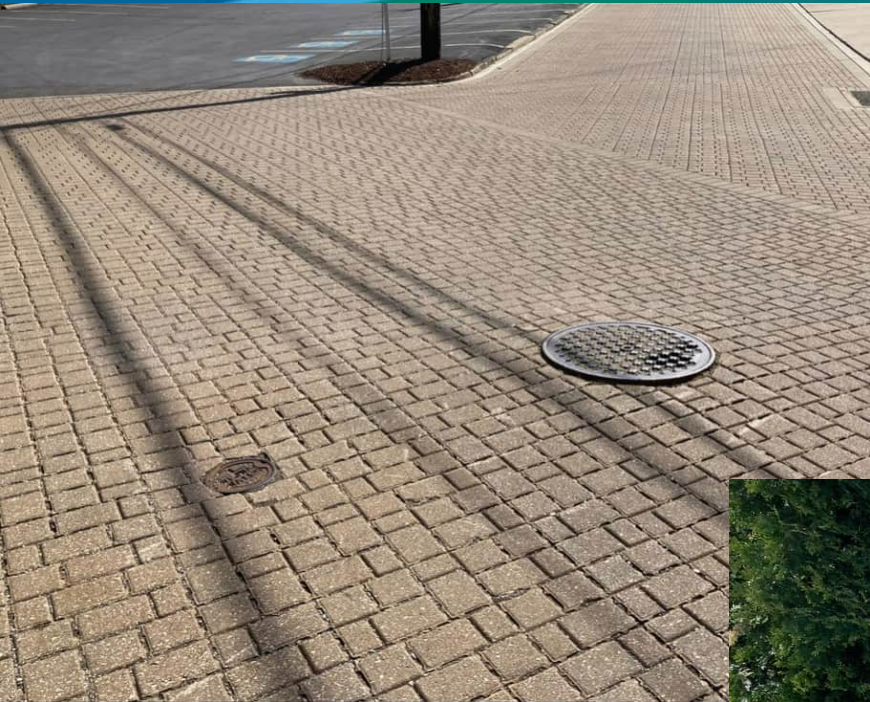
Pavers in good shape
